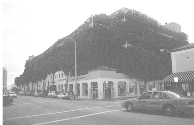
Fig. 14. South Beach, Miami. Planted trellis of Parking Garage contributes to reduction of urban heat island. SITE (James Wines) Design Architect.
